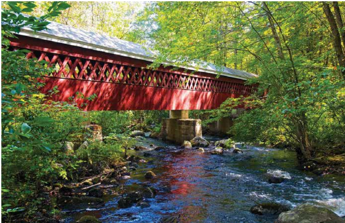
Pedestrian covered bridge over the Nissitissit River near Lake Potanipo in Brookline, NH. Photo: Ken Hartlage.
