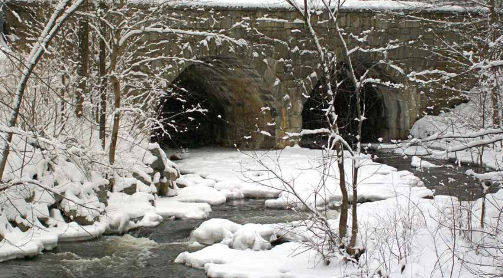
Bridge over Squannacook River. Photo: Kim King.
