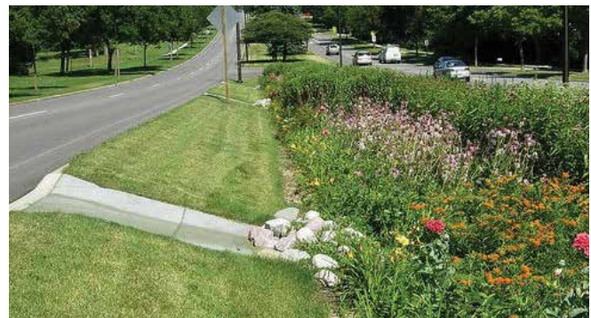
Example of rain garden used to filter road runoff. Photo: Aaron Volkening via Flickr Creative Commons License.
