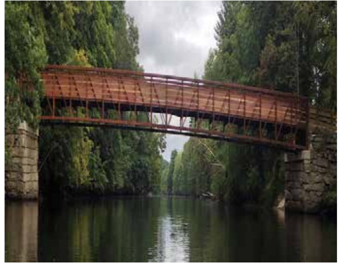
Current Fitch's Bridge in Groton, MA. This pedestrian-only bridge connects over 100 miles of trails that had been bisected by the Nashua River. Photo: www.freedomsway.org .
